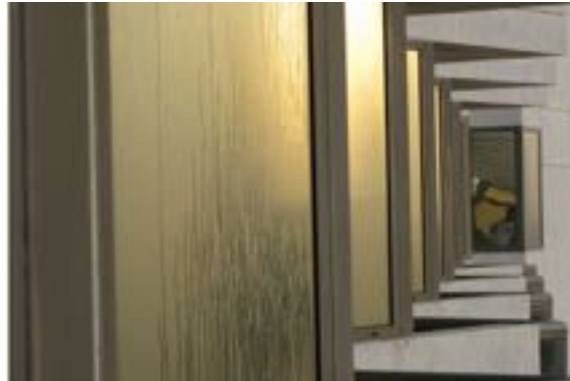
Typical morning condensation in the UAE, here at the Beach Rotana Hotel
