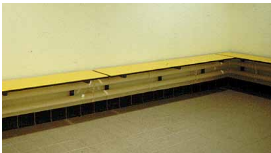
Cantilevered benches in a group changing room allow easy cleaning of the floor. A wall-hung heating source is located under the bench
