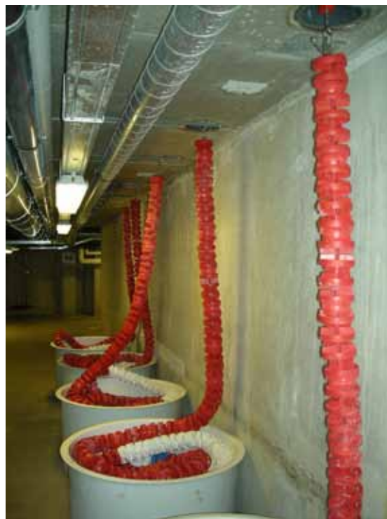
An alternative to storing lane ropes in a pool store – lane ropes can be stored in hoppers in the pool undercroft and accessed through stainless steel covers set into the pool end surround
