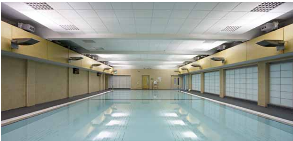
Well-designed uplighting can provide good overall illumination whilst achieving an attractive space. Avoid locating fittings above the pool unless accessible from a gantry
