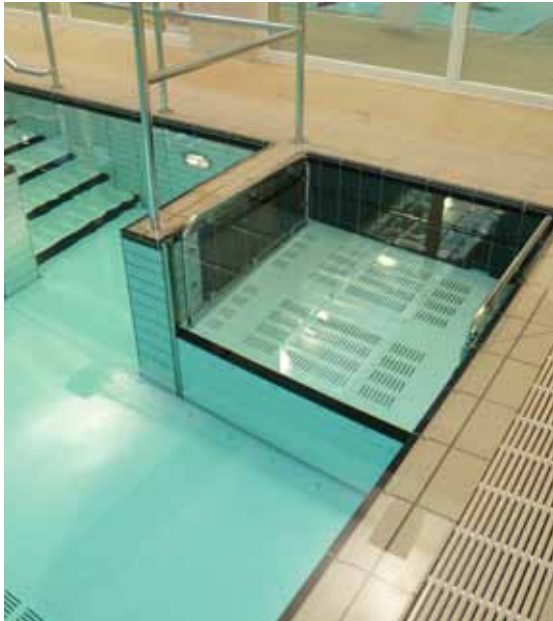
Submersible wheelchair lift and 'easy going' retractable steps integrated into a movable floor
