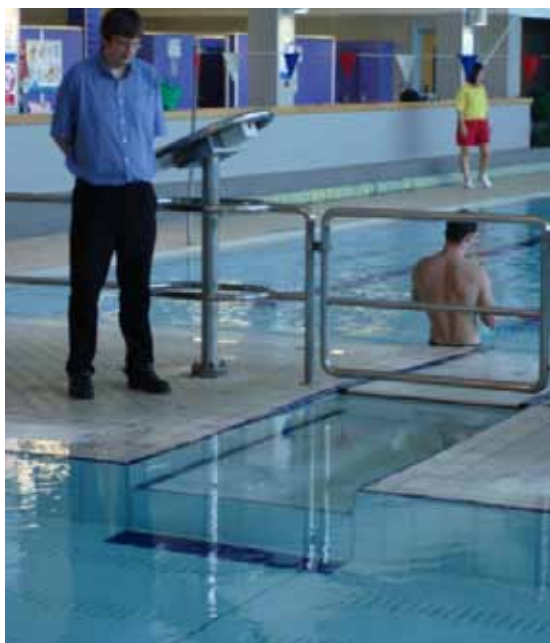
A submersible pool surround lift integrated into the pool as part of the pool surround can provide a dignified access to the pool for wheelchair users
