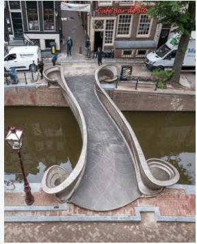
3D printed steel bridge, Amsterdams. Arup, MX3D, Joris Laarman Lab (2018)
