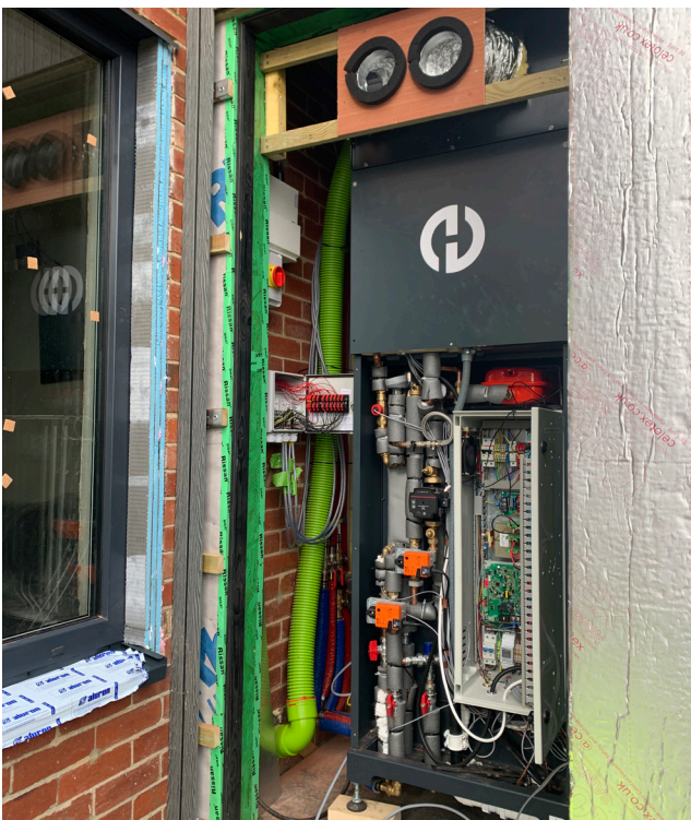
Ventive Home-B, a fully integrated 4-in-1 module: ventilation, heating, cooling and hot water system.
