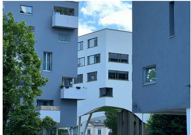
New buildings - Strubergasse neighborhood
