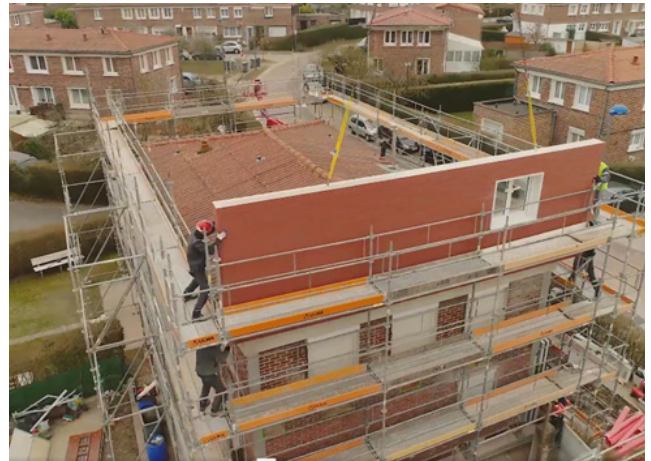
Step 4: On-site Integration and extensions of additional building elements.
