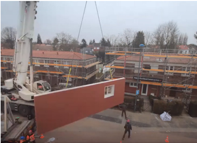
Step 3: On-site Integration and extensions of additional building elements.
