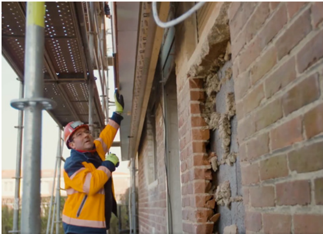
Step 5: The mounting of prefabricated modules exploring a new construction process.
