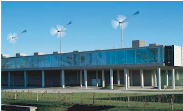
Fortis Montana WT - 5m diam. 15 – 18m high 2.5kW at 10m/s >> 5kW at 17m/s
