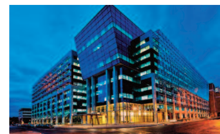
2016 CIBSE Building Performance Awards Winner: Sirius Building, Canberra, Australia (Mirvac Group)
