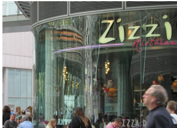
Figure 3.15: Excessive edge distortion due to the radial formed process.
