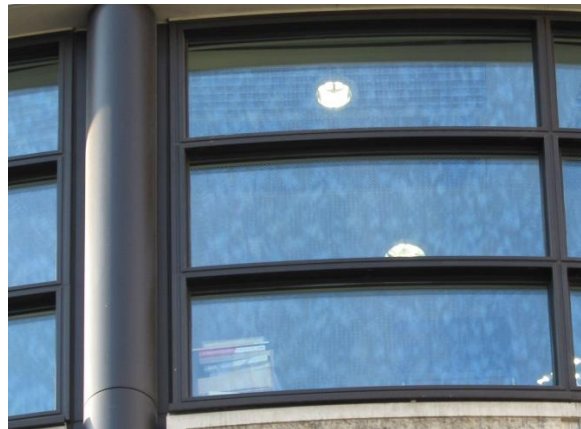
Figure 3.17: Anisotropy viewed due to tempering.
