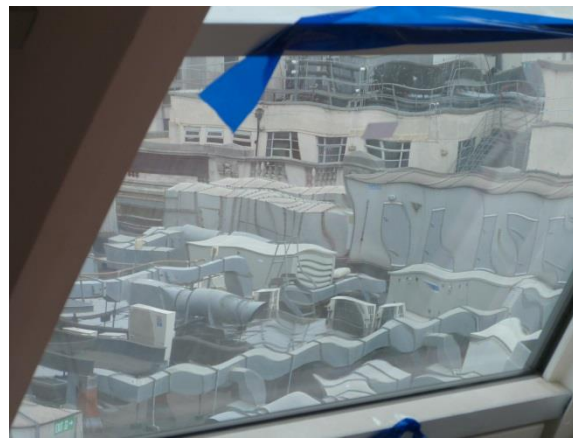
Figure 2.25: Lensing effect due to roller wave and multilayer glass lamination. (Ramboll, 2013)
