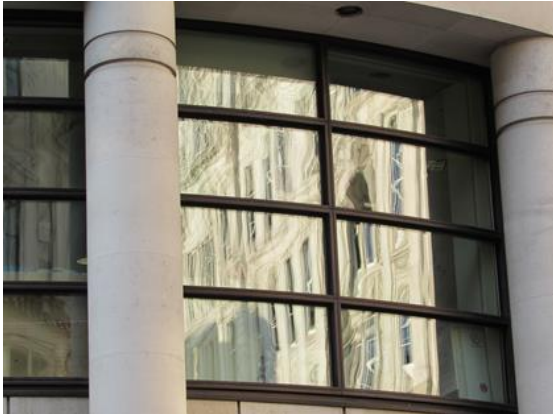
Figure 3.12: Distortions in the radial bent glass.
