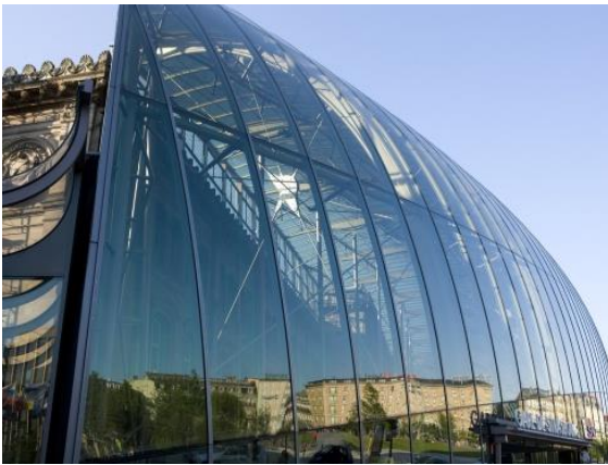
Figure 2.36: Strasbourg Station by Seele. (Open Buildings, 2015)
