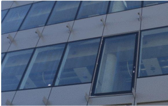
Figure 2.22: Contamination of rollers causes marks on the glass - white haze. (Ramboll 2013)
