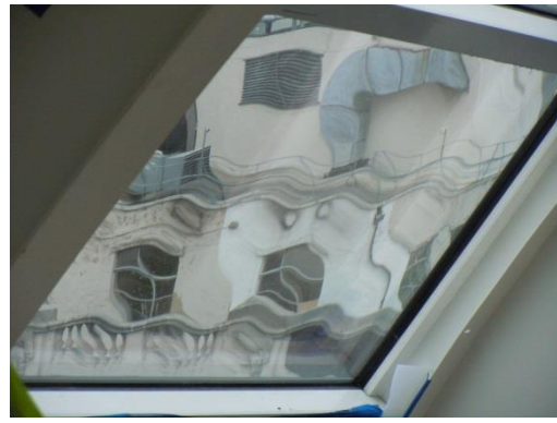
Figure 3.21: Anon project: Subsequent multilayer lens effect due to lamination and roller wave.
