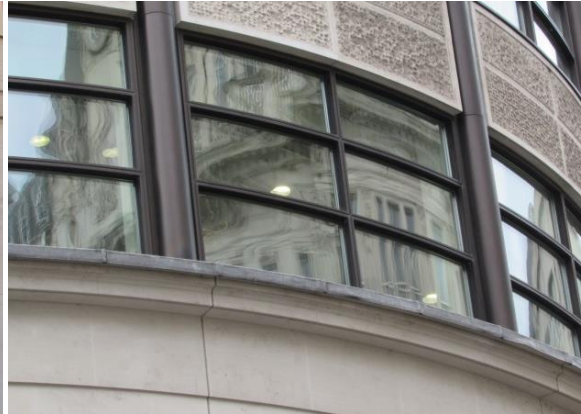
Figure 3.13: Distortions in the radial bent glass.
