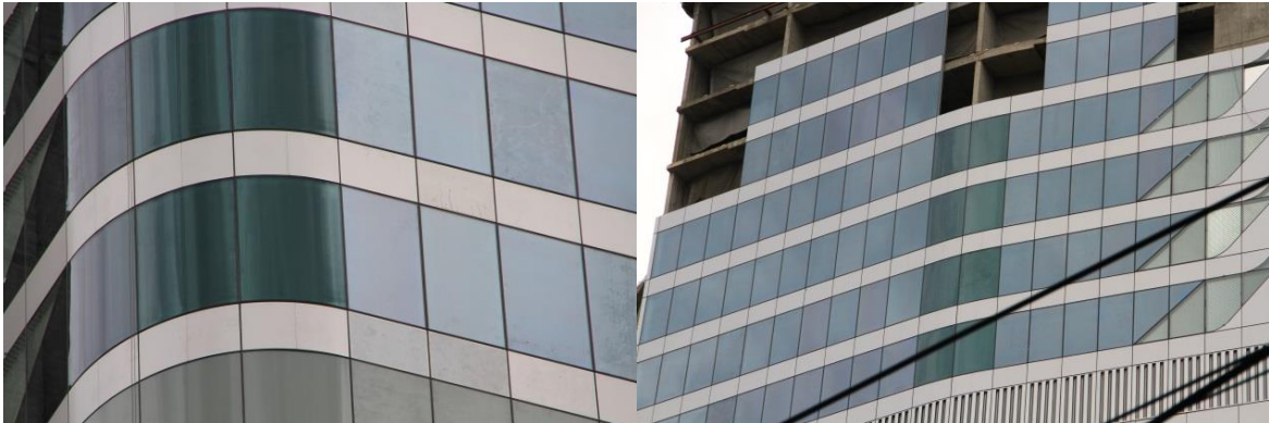
Figure 3.6: Coating inconsistency between the curved and flat glass. (MFT, 2015)
