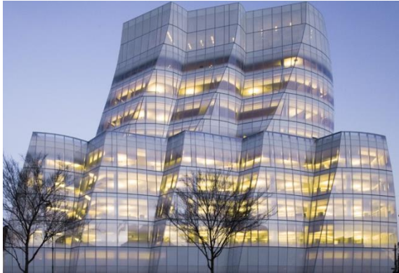
Figure 2.33: The Gehry designed IAC Building New York, USA. (Permasteelisagroup, 2015)
